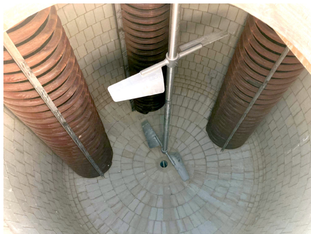
Figure 5. Brick-lined above-ground sulfur melting tank.
