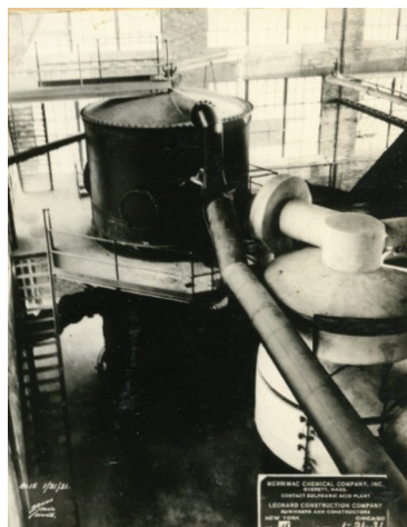
Fig. 1: Acquired by Monsanto Chemical Co. in 1930, the expanded capacity contact unit at the Merrimac Chemical Company plant in Everett, Mass, produced 75 STPD. These indoor units, built by Leonard Construction Co., operated with feed gas supplied by combustion of molten sulfur using contact units filled with T-210A catalyst.
