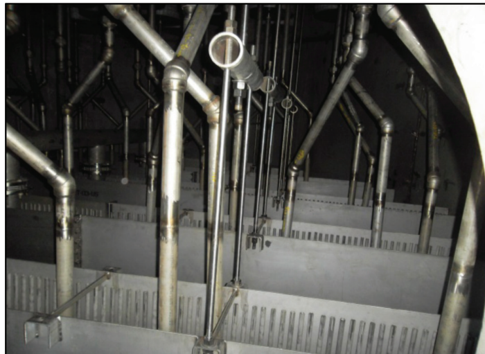
Fig. 6: Element seal legs routed to distributor troughs.
